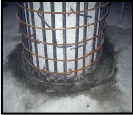
Fig 1.5: Structural Jacketing of a column
