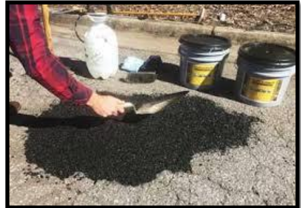
Fig 1.3: Flexible pavements require patching at times during their service life.
