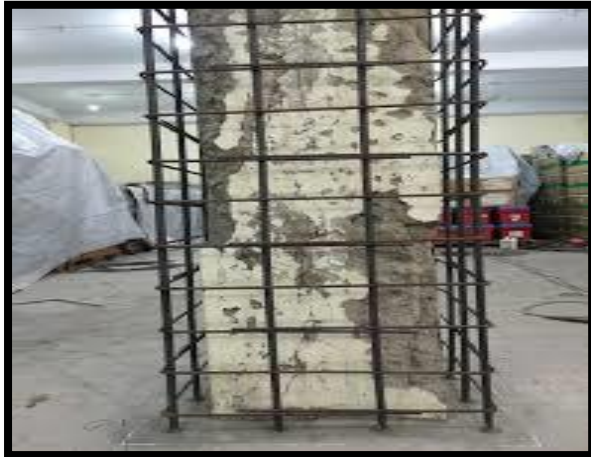
Fig 1.2: Concrete jacketing involves placing an additional layer of concrete around the existing columns.
