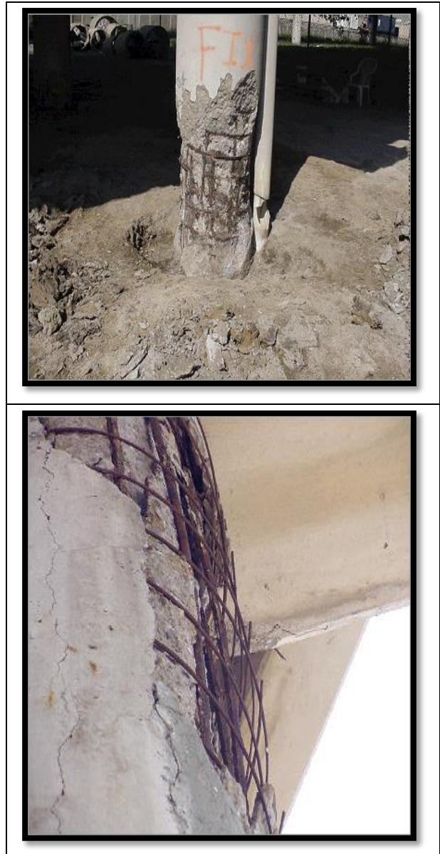
Fig 2.2: Sulphate attack on concrete is a chemical breakdown mechanism where sulphate ions attack components of the cement paste.
