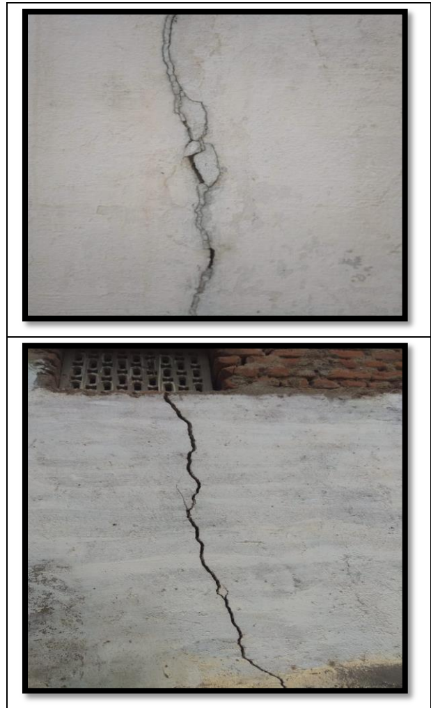
Fig 2.1: Non-structural cracks occur mostly due to internally induced stresses in building materials
