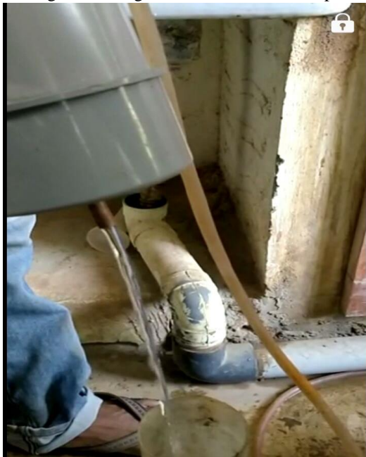
Fig. 3. Collecting discharge into the measuring jar
